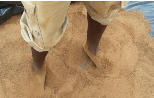
Mixing the dry sieved manure and the dry sieved clay
